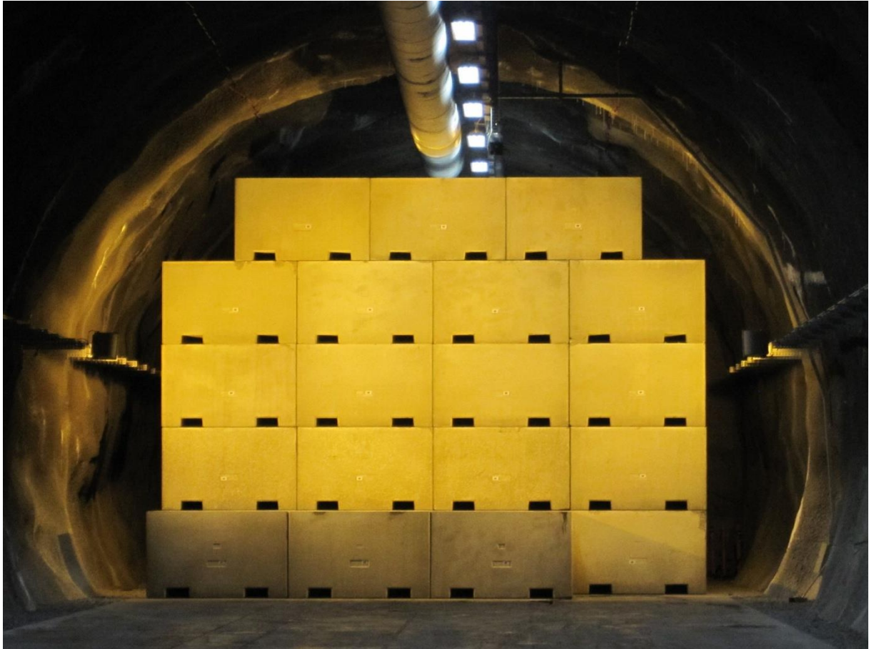
Figure B.2.1 – 3. Containers disposed in the I-K1 vault of the National Radioactive Waste Repository
