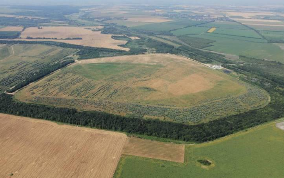
Figure An7.3 - 8: Remedied uranium industry tailings pond
