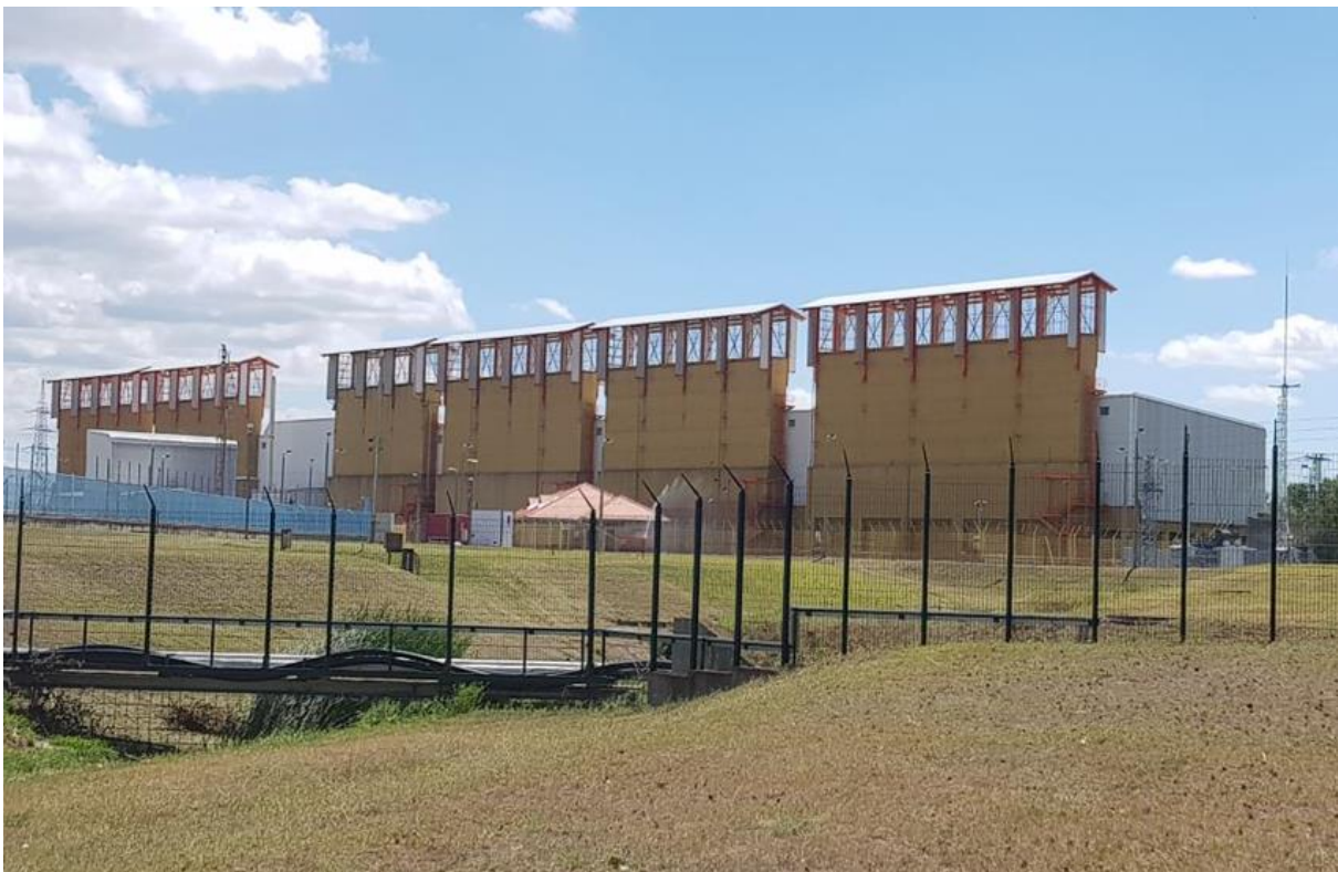
Figure G.1 – 1. Spent Fuel Interim Storage Facility
