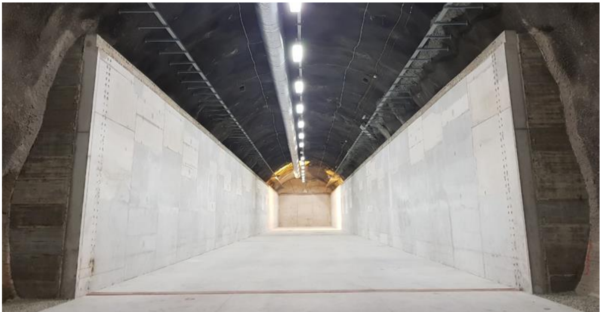
Figure H.3 – 4. Reinforced concrete vault in disposal chamber I-K2 of the National Radioactive Waste Repository
