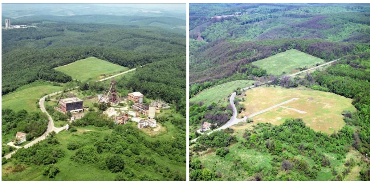
Figure An7.2.4-1: Air shaft IV of the uranium ore mine during operation and after remediation
