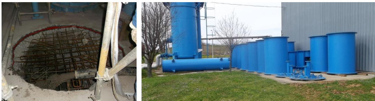
Figure An7.3 – 2: Expansion of the water treatment system in pictures
