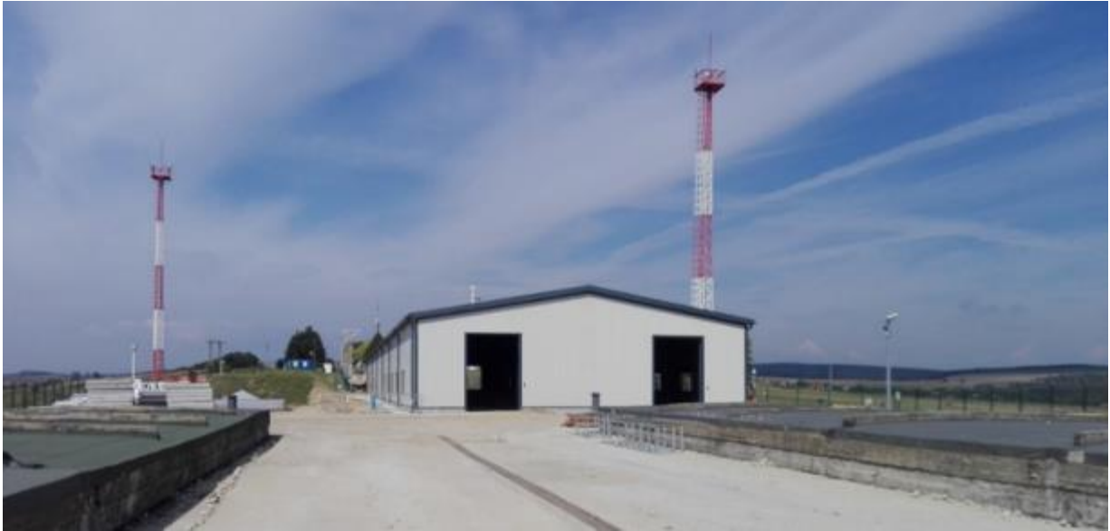
Figure K.3 – 3. Light structure hall over the vault row 1 in the RWTDF
