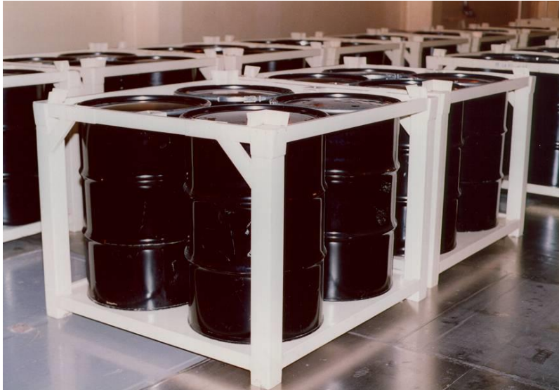
Figure D.2.4 – 3. Storage of low and intermediate level waste
