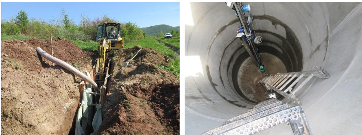
Figure An7.3 – 5: Construction of the drain leakages system of the dumps
