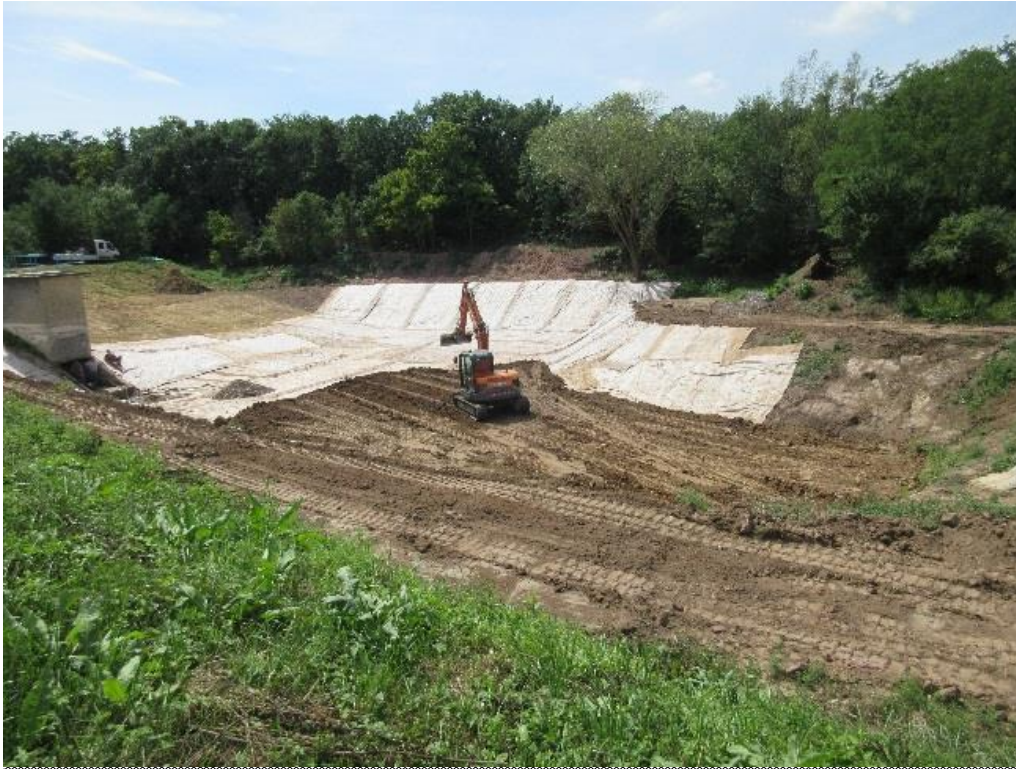
Figure An7.3 – 6: Construction of emergency mine water reservoir
