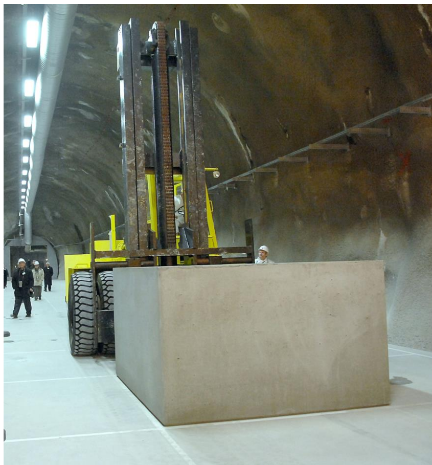
Figure H.3 – 2. Disposal of the first reinforced concrete container in the National Radioactive Waste Repository
